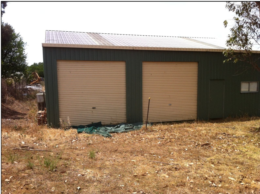
Plate 8 – Corrugated metal shed at Location 15.
