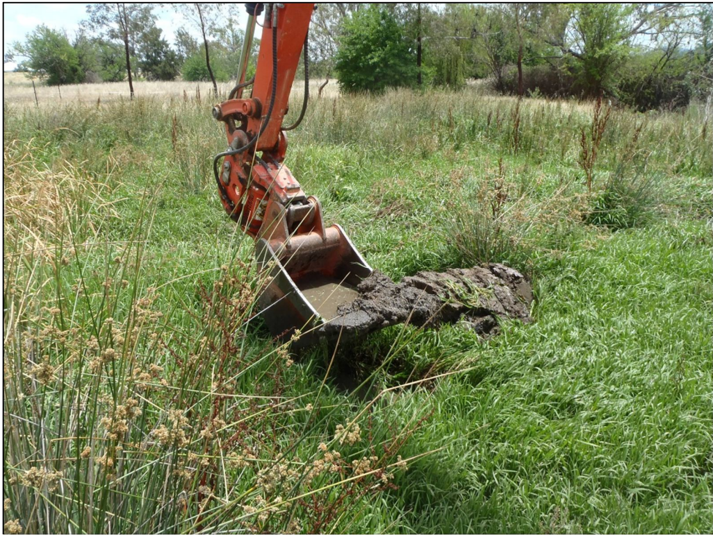
Plate 21 – Concrete and asphalt observed dumped in Barnes Gulley in the northeast portion of the site.
