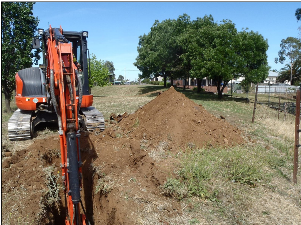
Plate 18 – Excavating fill materials on the northern portion of the Tamworth Bridge Club.
