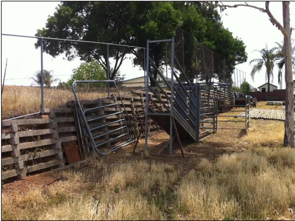
Plate 9 – Retaining wall along the northern boundary of the Tamworth Bridge Club property.
