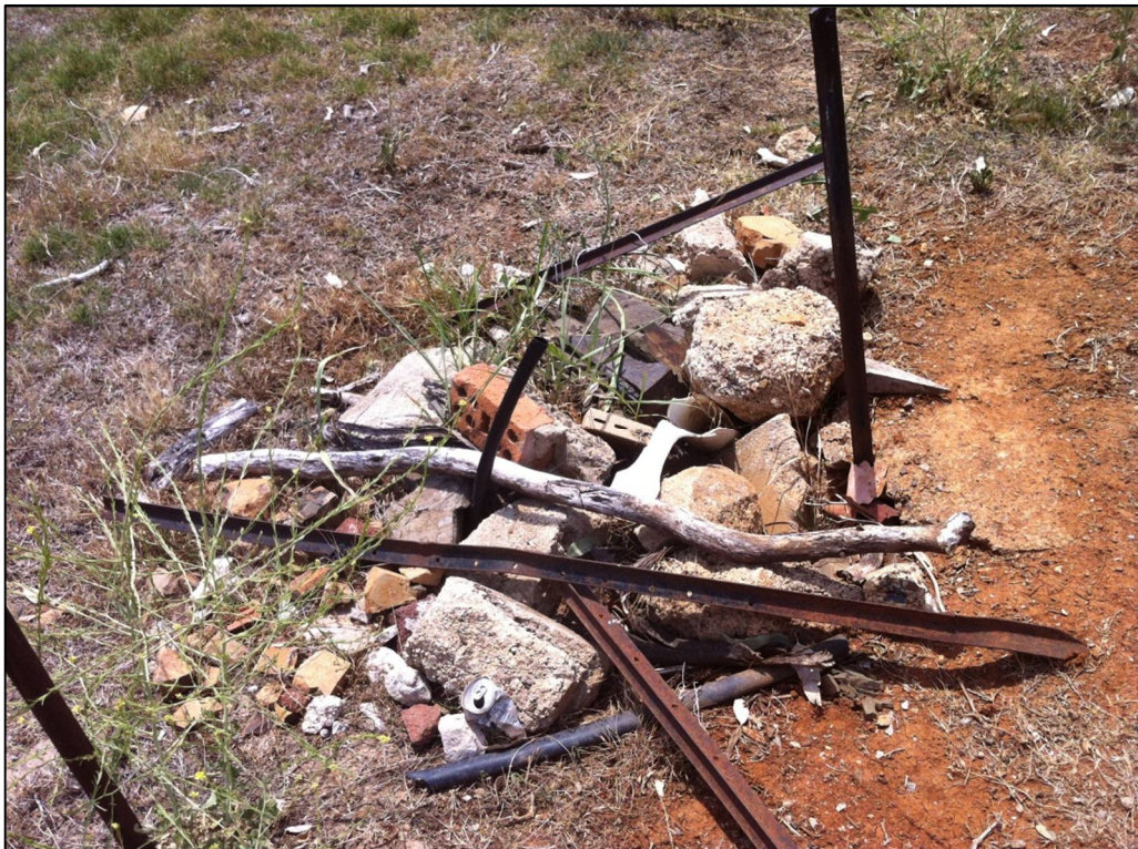
Plate 10 – Location 18, rubble filled in area.
