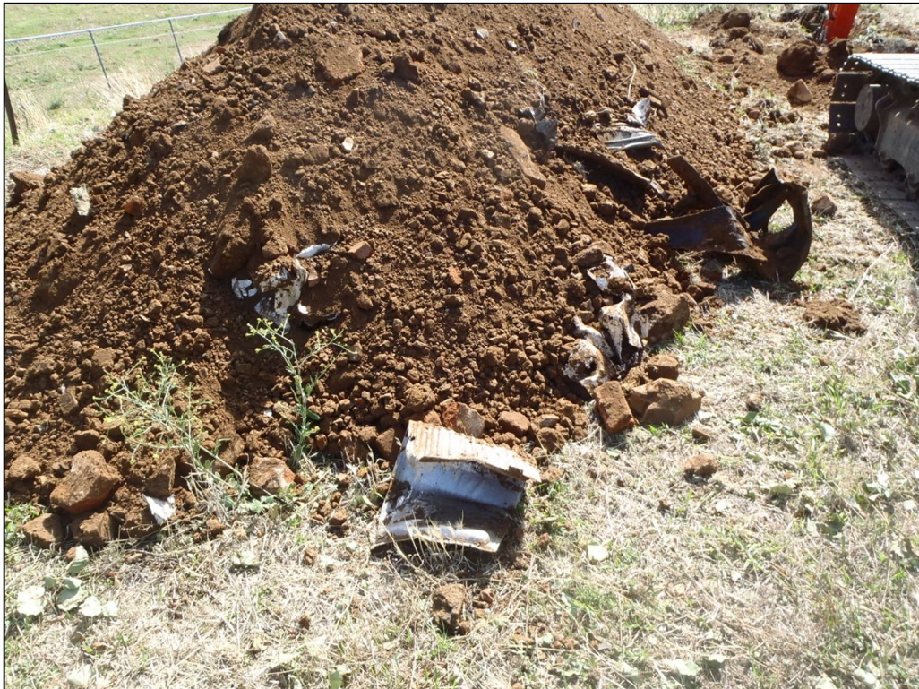
Plate 17 – Rubbish materials observed in fill material on the Tamworth Bridge Club.
