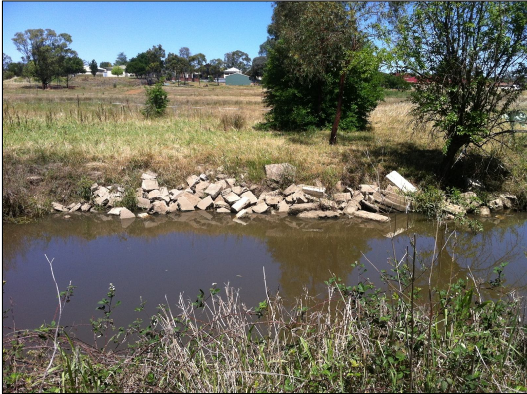
Plate 13 – Concrete dumped within Barnes Gully at the northeast corner of the site.
